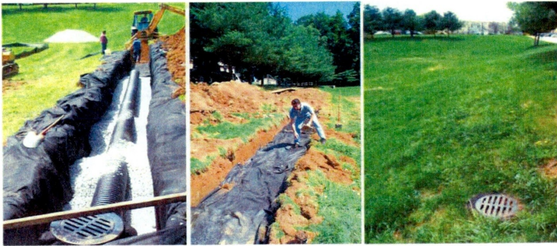
Figure 4: Example of Infiltration Trench Installation Source: PA BMP Guidance Manual, Chapter 6, Page 46.
